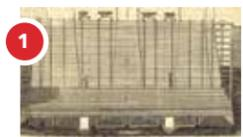
**1** Caissons form the foundation of the two bridge towers. Caissons Committee students research the science behind the watertight structures and construct the foundation.
